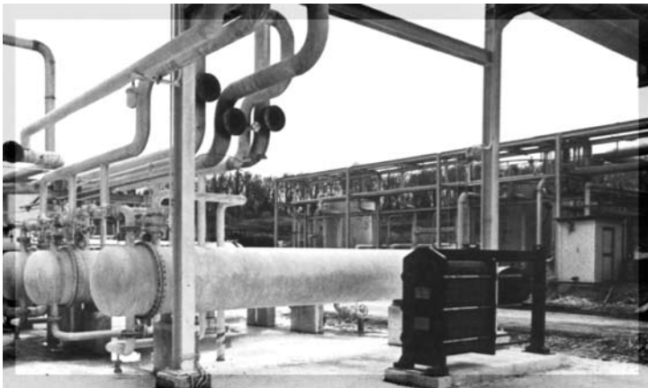
Figure 30. Picture of Series R405 Paraflow being installed.
