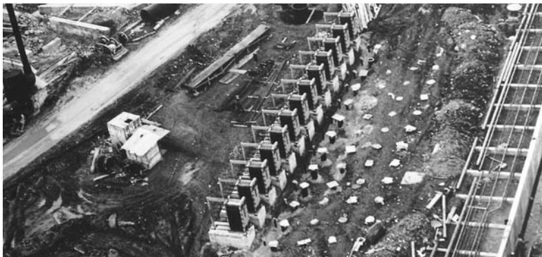
Figure 38. Ammonia/urea fertilizer plant under construction with 13 plate heat exchangers as central coolers.
