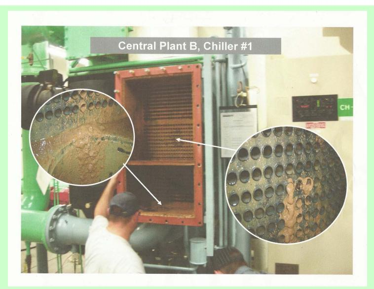
Cooling tower systems become incubators for biogrowth, fouling, under deposit corrosion
